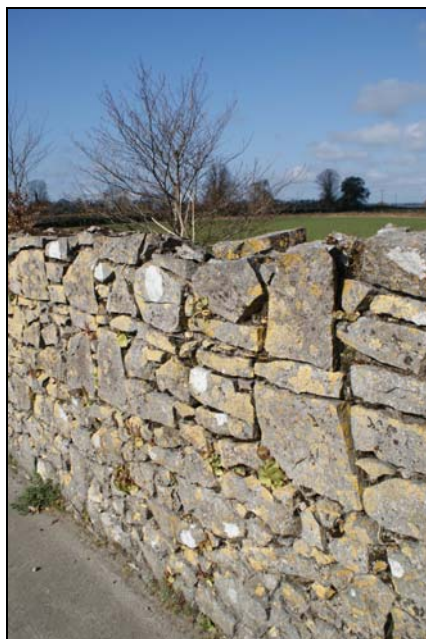
Plate 6. Stone wall along the road entering Johnstown from the south west.
