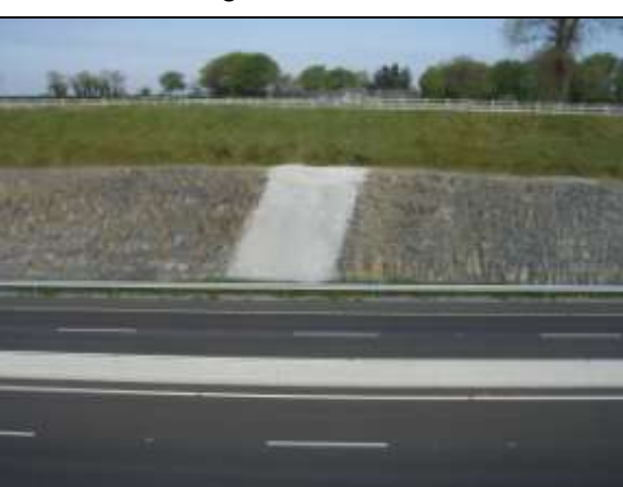
Concrete patch over weak ground.
