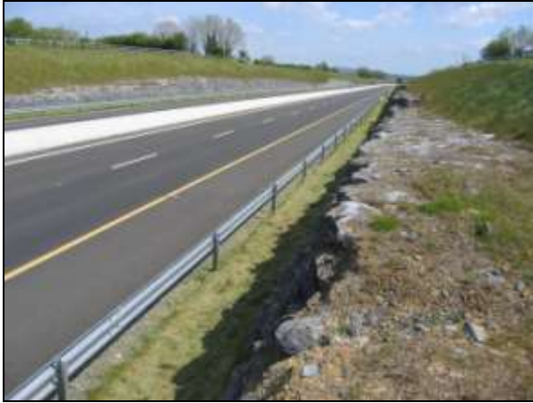
The cutting looking north on the east side.
