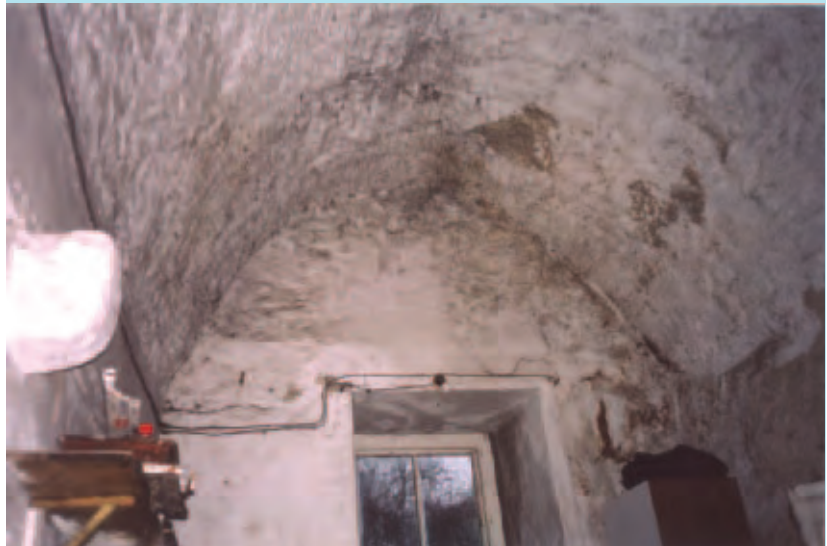
Plate 25: Black Rath's Castle: Vault with wattle shuttering
