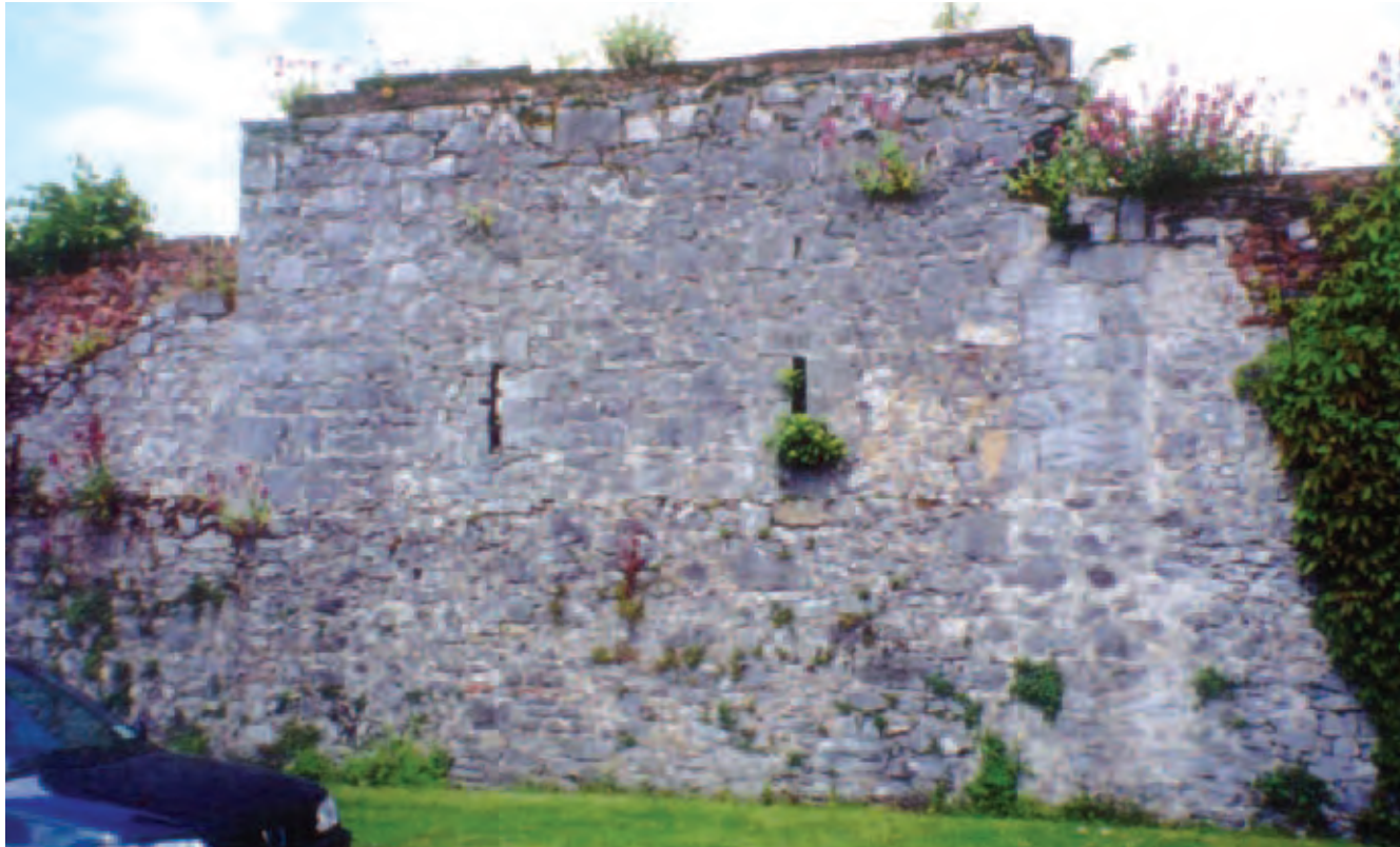
Plate 31: Section of wall displaying two loops, located to south of Langton's Bar (June 2001)
